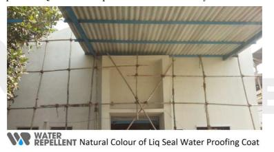
All cementations waterproofing sealing slurries or membranes have to be applied in such a way that after drying a layer with a thickness of at least 2 mm will result. This is generally obtained only with multiple coating, mostly with two or three coats (typical drying time is 2 to 5 hours before application of the second layer).
